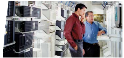
Can be integrated into high density racks.
